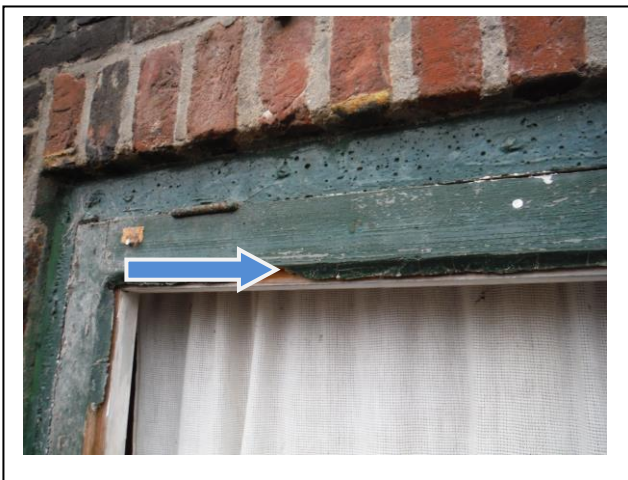
Foto 10: M4: Stopverf, beglazing
