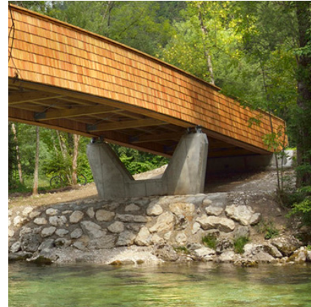
Slope under bridge
